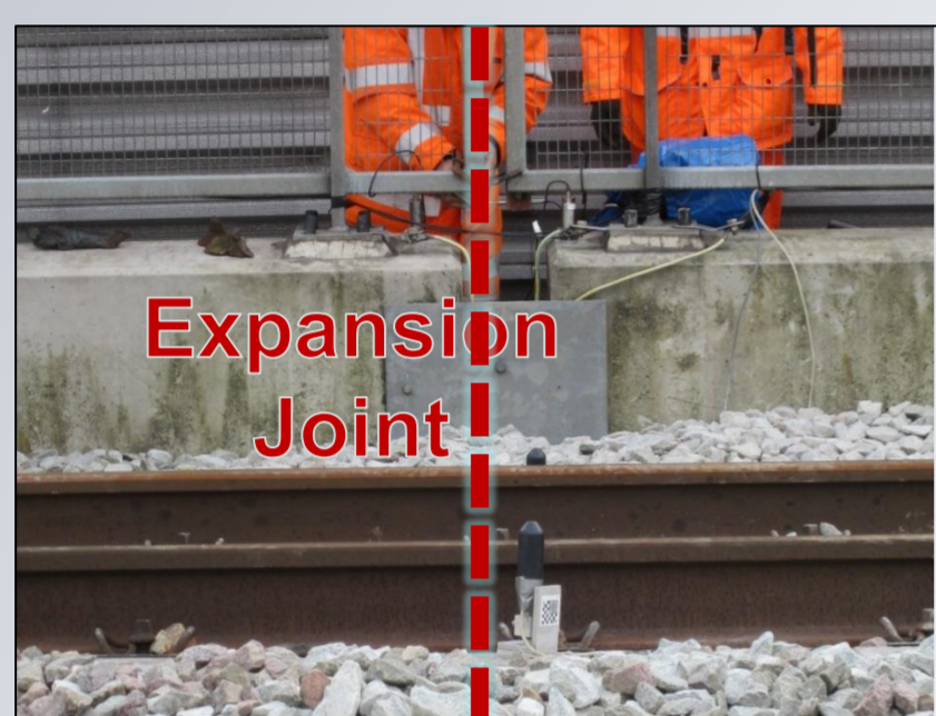
Figure 2 – Expansion joint
